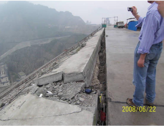
图2 四川省紫坪铺大型水库坝体背水面出现数条裂缝、垒石受挤压向外凸出、坝体整体下沉约20cm Fig. 2 Fractures, upward-projecting of rocks and subsidence of 20cm in the dam of Zipingpu reservoir.
