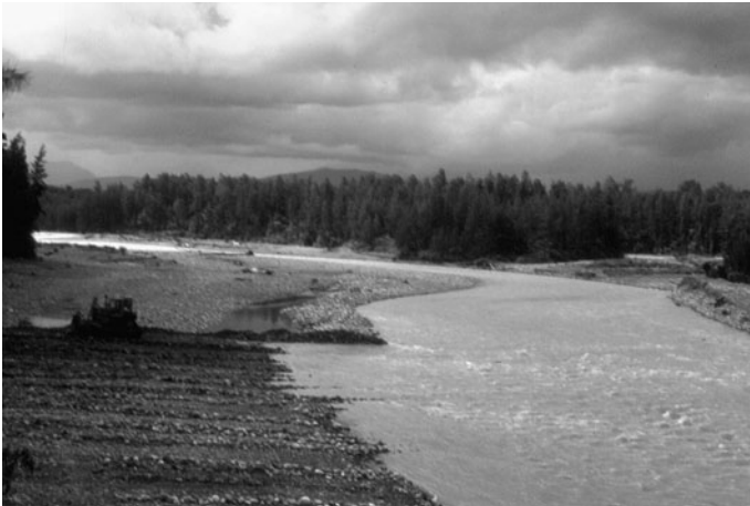
Fig. 4.14 Earthworks in the Ajkwa River, Irian Jaya, Indonesia. Tailings are discharged (~8.7 Mt per year) from the giant Grasberg-Ertsberg mine into the Ajkwa River, causing severe aggradation and flooding of vegetated lowland downstream of the mine. Areas inundated with tailings are to be turned into productive and sustainable agricultural land
