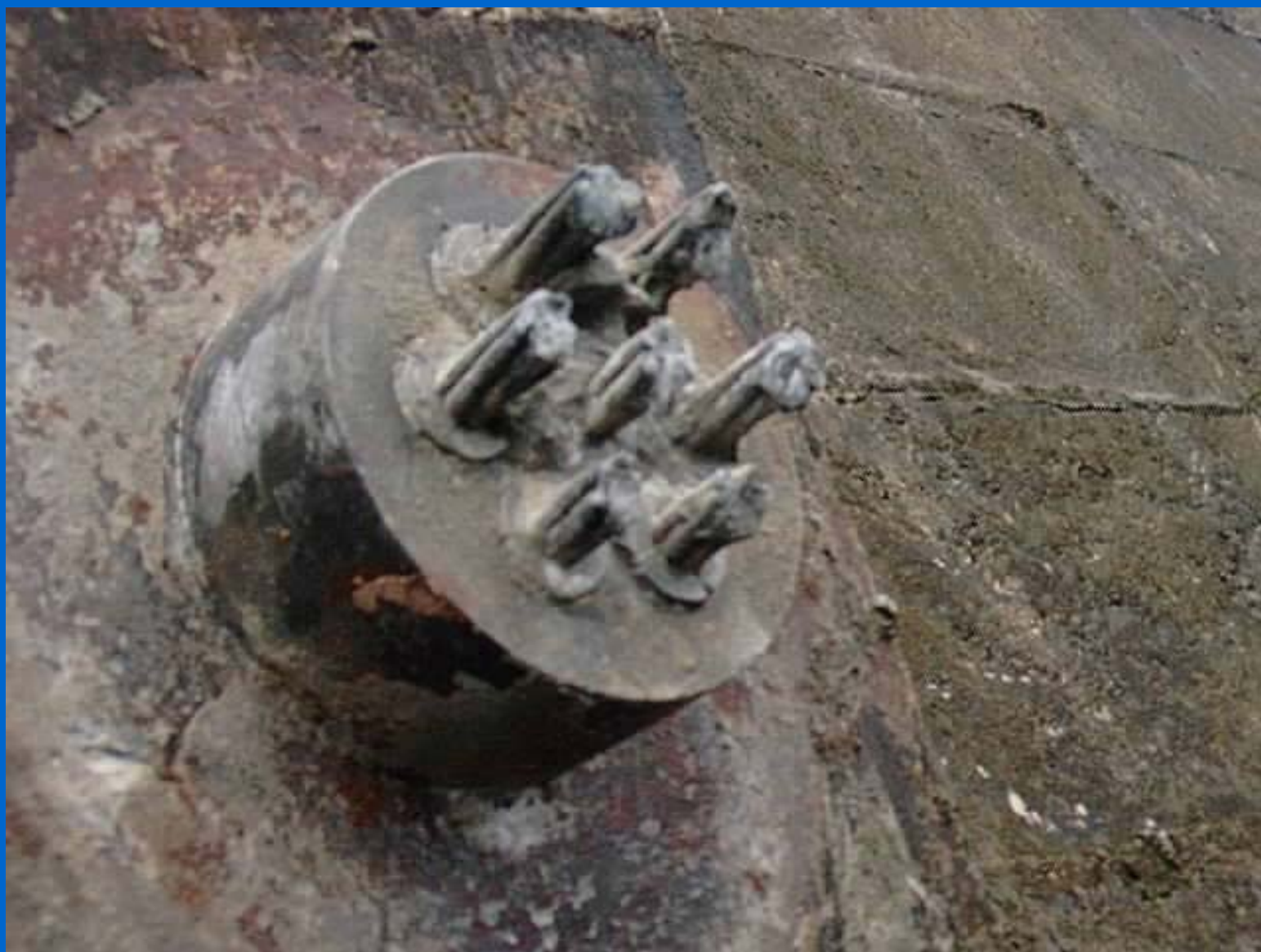
凿开后锚具及钢绞线的锈蚀
