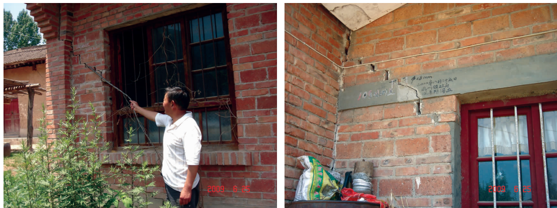
图 4 滑坡体上房屋出现裂缝 Fig. 4 Cracks in houses on the landslide body
