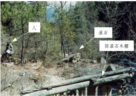
图 8 棚顶滚落的 20 多个滚石(最大直径约 2 m) Fig.8 More than 20 rockfalls on the roof of wood shed (the biggest one is about 2 m diameter)
