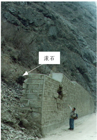
图 4 84~85 道班一滚石击穿 1 m 多厚的石砌挡土墙 Fig.4 Stone-built retaining wall 1 m thick, hit by one rockfall between squad 84 and 85
