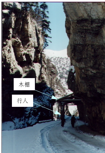
图 1 80 道班南侧的陡崖段(II d1 )及防滚石木棚 Fig.1 Steep cliff (II d1 ) and wood shed against rockfall at squad 80
