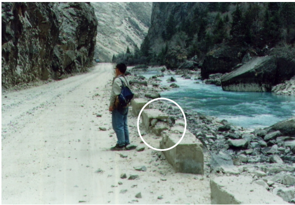
图 3 84~85 道班被滚石砸坏的混凝土护墩 Fig.3 Concrete piers damaged by rockfall between squad 84 and 85
