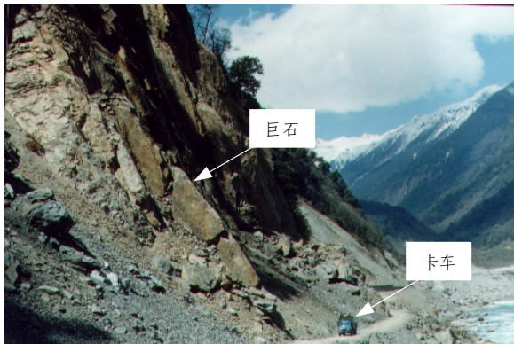
图 7 大老虎嘴北侧岩石崩塌体斜坡(VI x1 ) Fig.7 Slope (VI x1 ) with rock blocks distributed at north of Dalaohuzui bend
