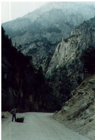
图 5 85~86 道班路面上一个滚石(尺寸约 1.0 m×0.7 m×0.5 m) Fig.5 One rockfall on road (about 1.0 m×0.7 m×0.5 m) between squad 85 and 86
