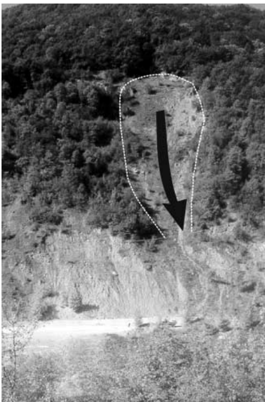
Fig. 3 General view of an identified landslide in the area
